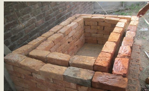
zero-energy evaporative cooler
